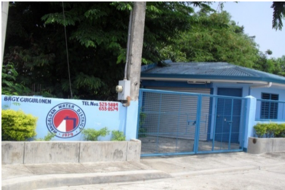
Pumping Station at Brgy. Guiguilonen
