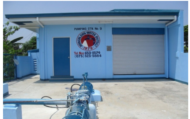
Pumping Station at Brgy. Bari
