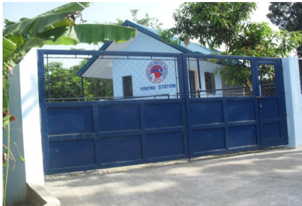
Pumping Station at Brgy. Salay (NEW)
