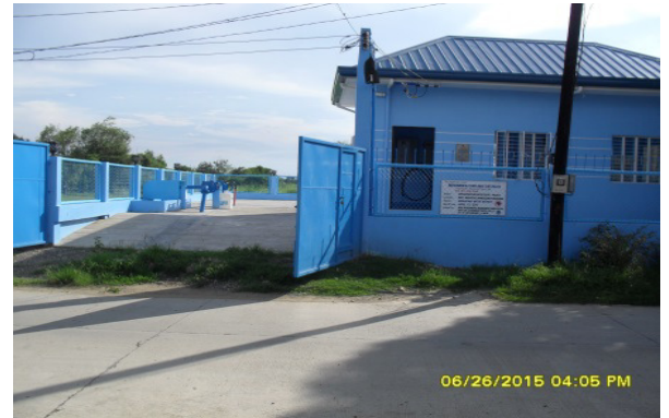
Pumping Station at Brgy. Macayug
